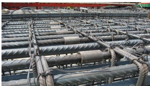
Fig -2: Coupler on site
