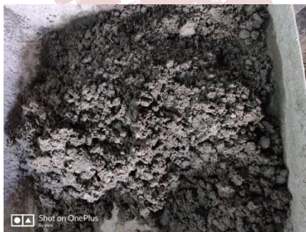
Mixing of concrete
